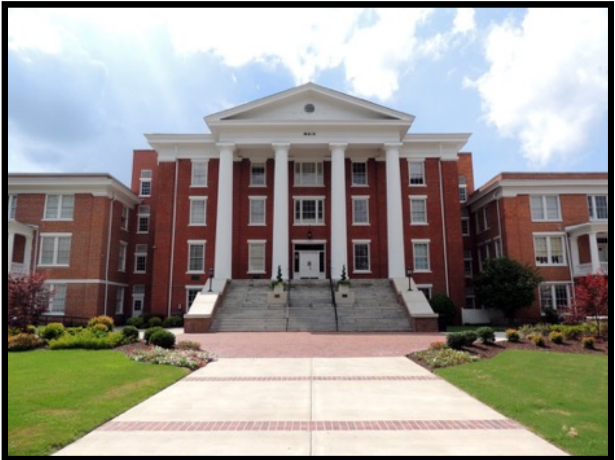
Main Building. Louisburg College, Louisburg, North Carolina.
